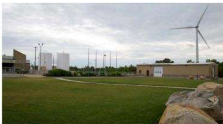
Figure 20. Wind project on Joint Base Cape Cod. Photo from U.S. Air Force
