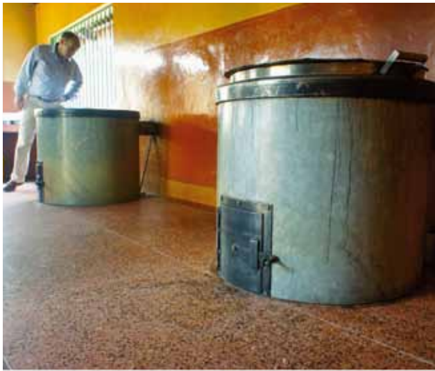
Kitchen at women's prison Shimo la Tewa after refurbishment
