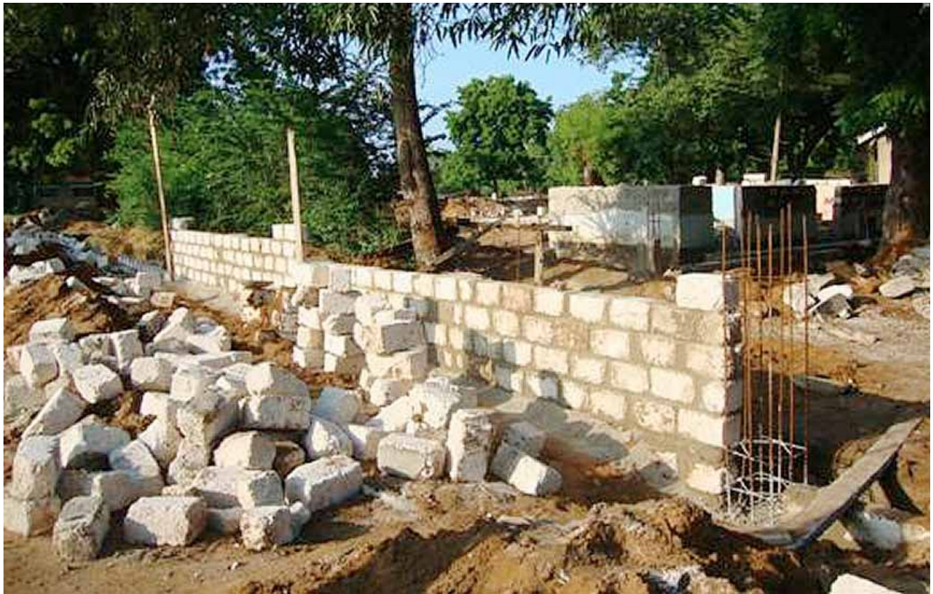
Shimo La Tewa Courtroom construction in progress, May 2010
