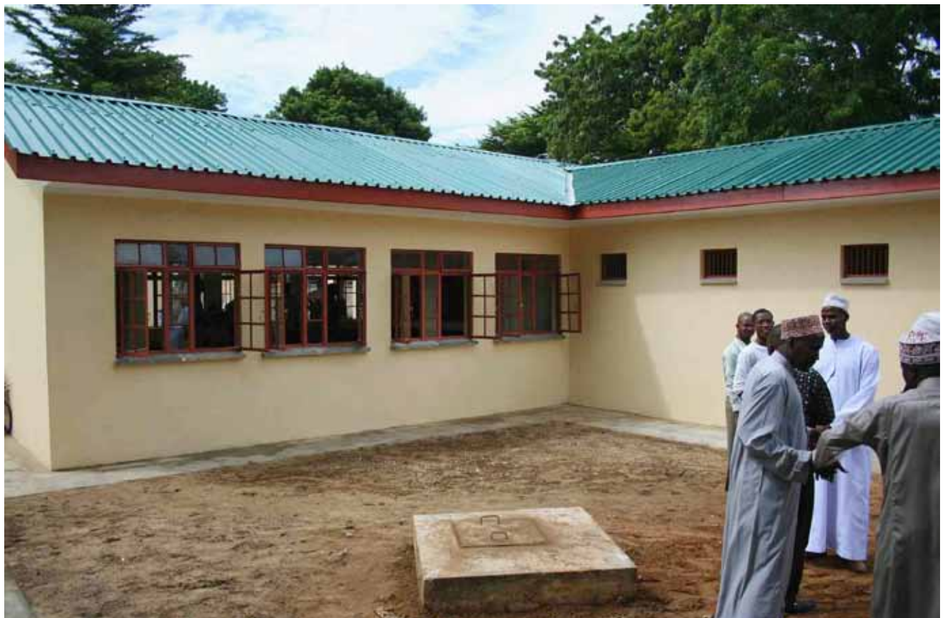
Newly refurbished Shimo La Tewa Court Room, June 2010
